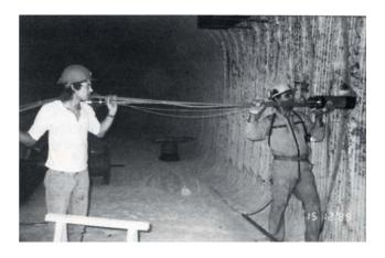
The preadjustment of the displacement transducers is done by expansion anchors by which also the compound of anchor-rock is ensured. These works are carried out by settlement rods from borehole mouth to any installation direction.
