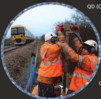
QD (Quick Drive) Casing is an ABS inclinometer casing manufactured using advanced extrusion techniques.
