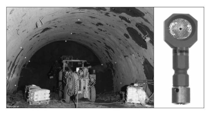
As fixing device, standard measuring bolts with a thread 3/8" are used which are either conventionally injected or subsequently drilled and solidified or are welded on the arch.
